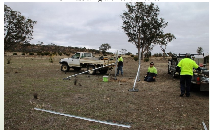
Green Army team helping to erect an enclosure
